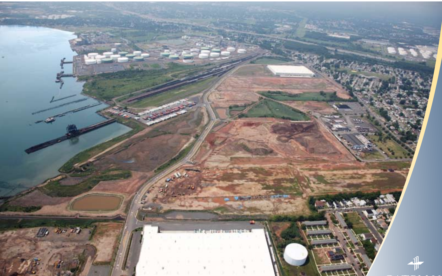
Port Reading aerial view of Newark Bay.
